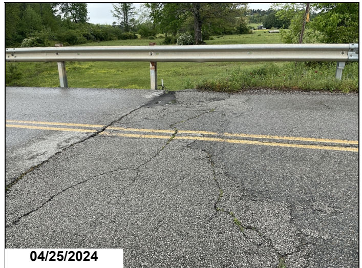
Abutment 1, Right, Approach Roadway: settlement causing a 4' X 3' pothole.
