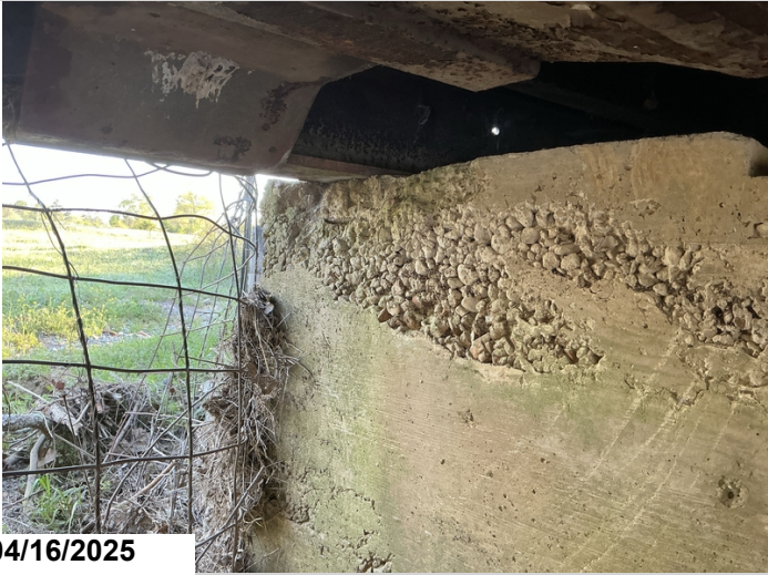
Abutment 1, Right Railcar, Girder 8: spalling with exposed reinforcing steel. No Section Loss.
