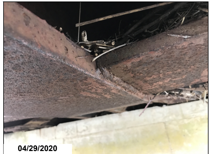
Right Railcar has Broken weld to brace plate welded between Girders and 6 & 7 @ 3/4 point.
