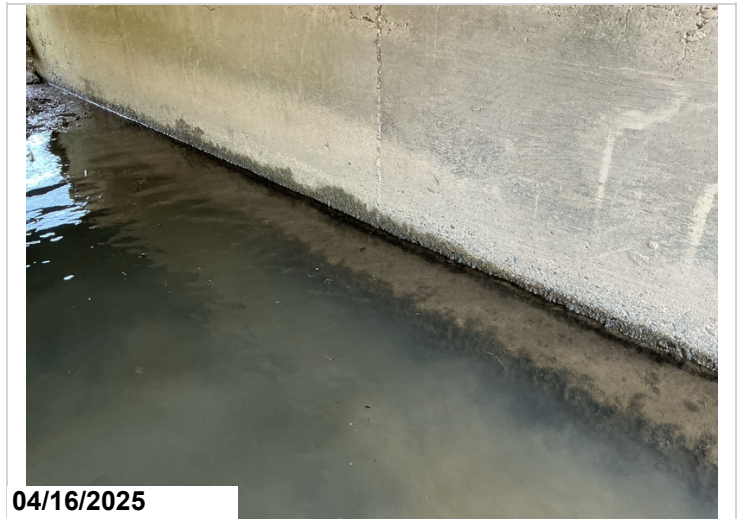
Abutment 1: footing exposed.(Footing is on solid rock)
