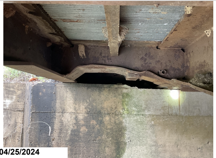
Left Railcar, between Girders 1 & 2, Bolster near Abutment 2: out-of-plane bending to cross member.
