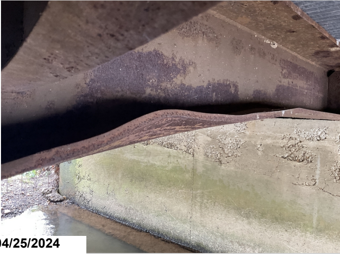
Left Railcar, Girder 4, Bottom Flange, 5' ahead of Abutment 1: twisted for 7'.
