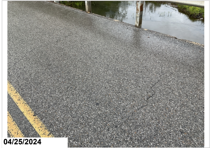
Deck: transverse cracking to asphalt overlay.
