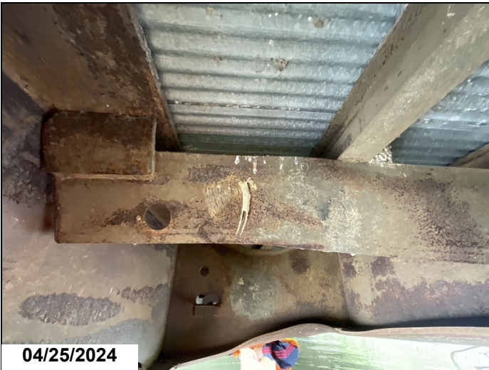
Cross brace, Back side of Floor Beam 1, between Girders 3 & 4: twisted.
