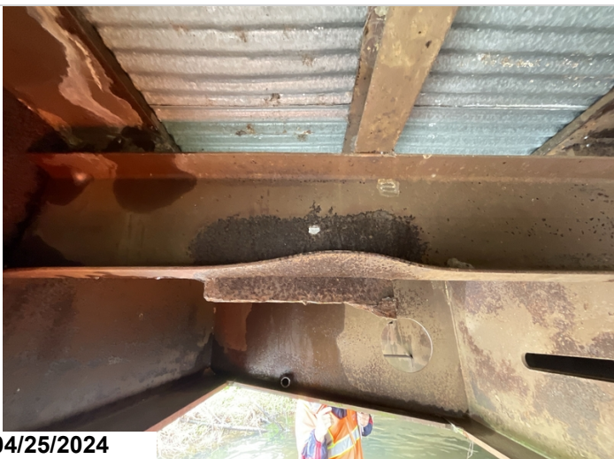
Left Railcar, Crosstie 2, between Girders 1 & 2, between Floor Beams 2 & 3: out-of-plane bending.
