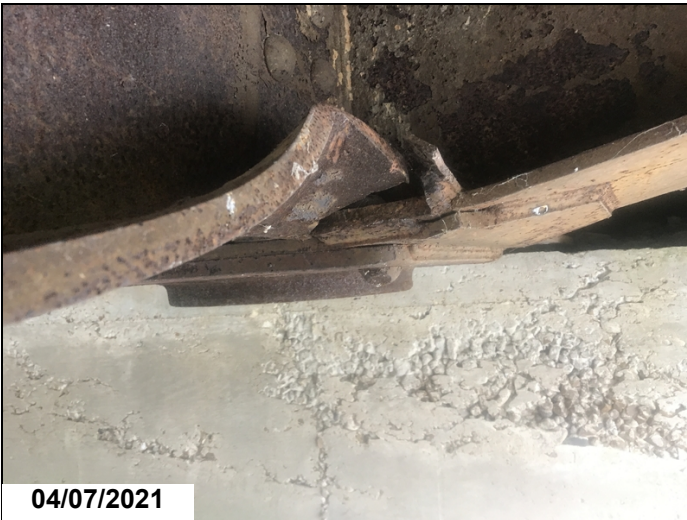
Longitudinal Girder 2 has 6" crack to bottom flange, and 1" vertical crack to web at Bolster near Abutment 1.
