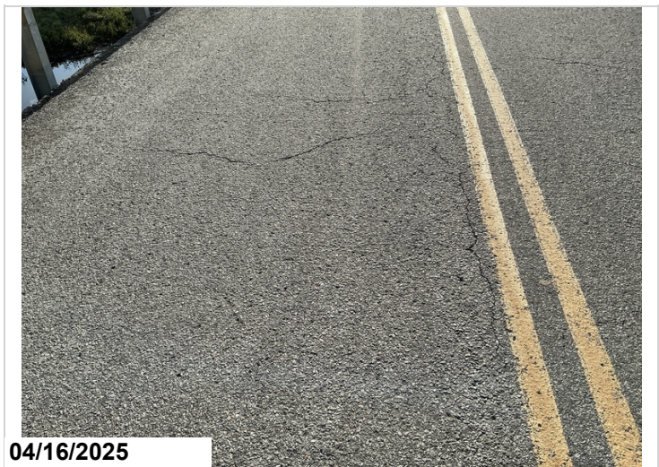
Deck: cracking to asphalt overlay.
