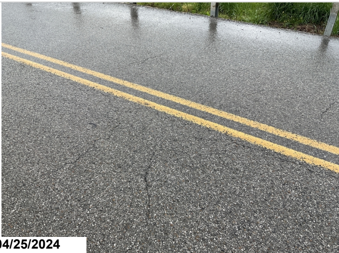
Deck: cracking to asphalt overlay.
