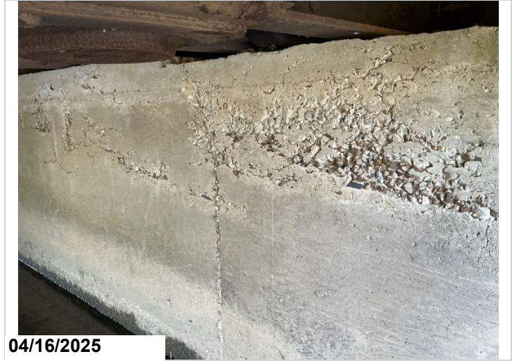
Honeycomb area to abutment 1.
