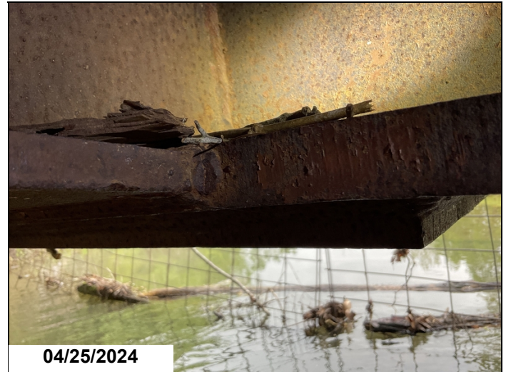
Right Railcar, Floor Beam 3, Left side of Girder 6: cracked weld.
