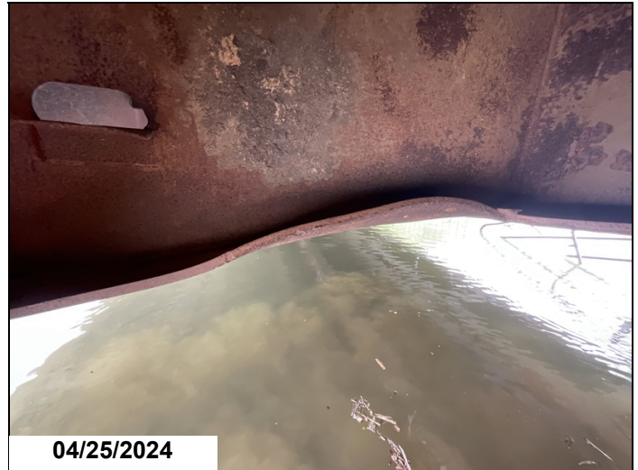
Floor Beam 1, Back, between Girders 3 & 4: out-of-plane bending.
