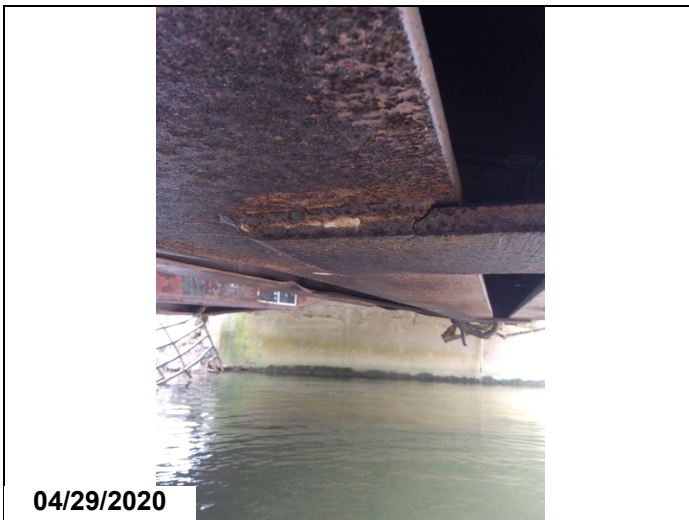
Typical broken welds and cracks to brace plate between Girders 2 & 3 on Left car.
