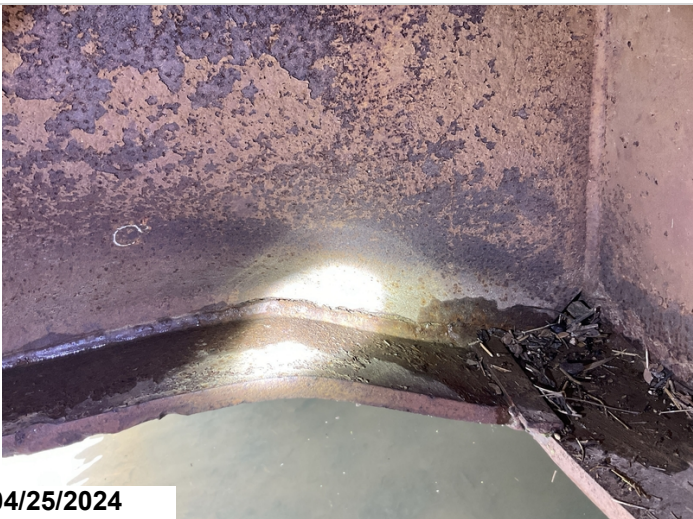
Left Railcar, Floor beam 1, Left side of Girder 2: crack along the web & bottom flange connection along Floor beam.
