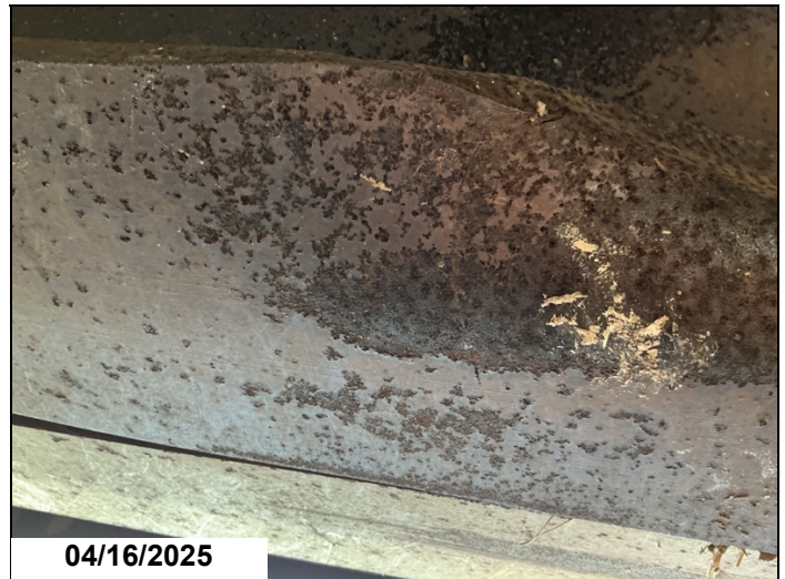
Left Railcar, Abutment 1, girder 3: 5" crack to bottom flange and large bent area 4.5' ahead of Bolster near Abutment 1.
