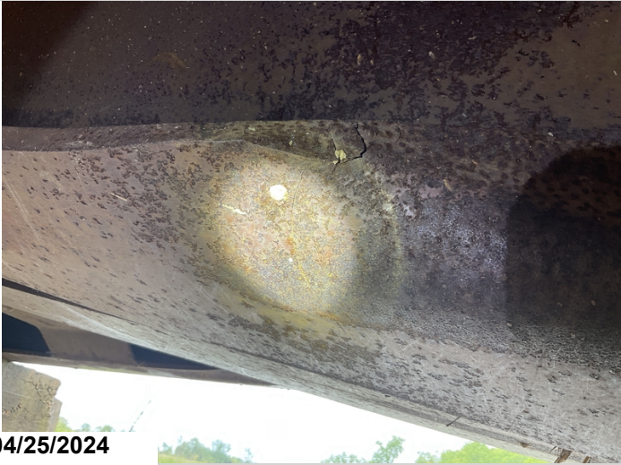
Left Railcar, Abutment 1, girder 3: 5" crack to bottom flange in large bent area 4.5' ahead of Bolster near Abutment 1.
