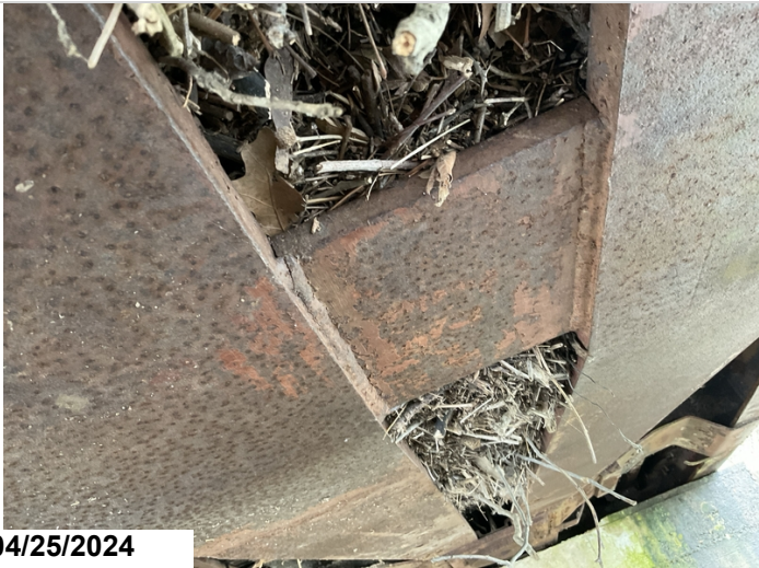
Right Railcar, Brace Plate between Girders 6 & 7: cracked weld near 3/4 point.
