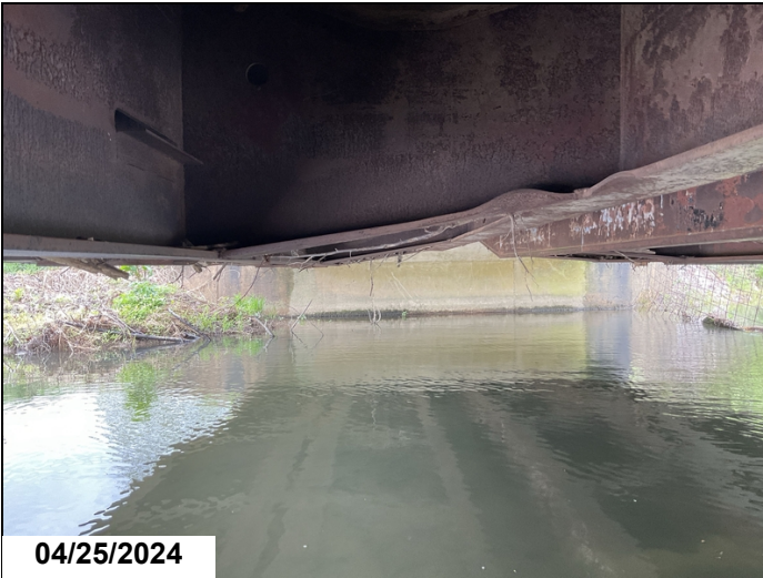
Floor Beam 2, Back, between Girders 3 & 4: out-of-plane bending.
