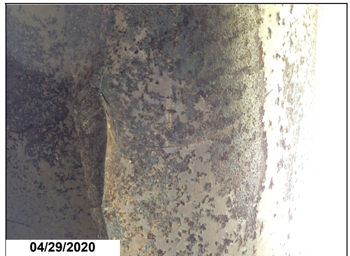
Longitudinal Girder 3 has crack in bottom flange where bent.
