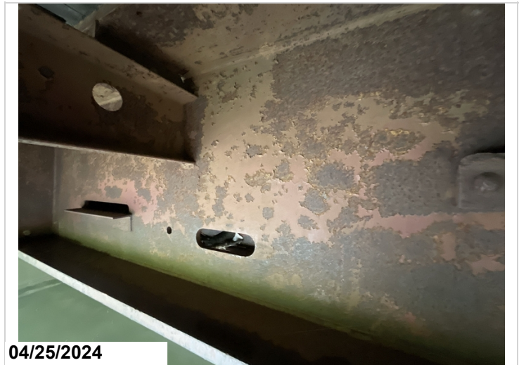
Typical flaking paint & surface corrosion.
