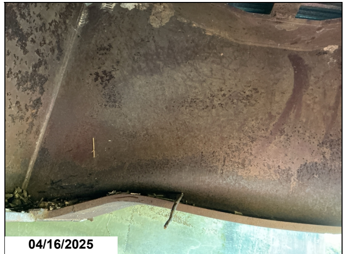
Left Railcar, Floor Beams 1 & 2, between Girders 3 & 4: out-of-plane bending to the bottom flange.
