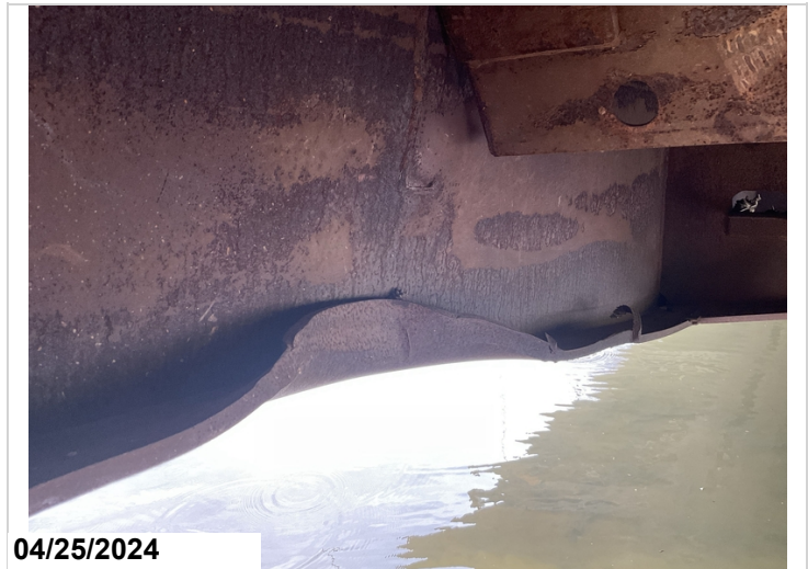
Left Railcar, Abutment 1, girder 3: 5" crack to bottom flange in large bent area 4.5' ahead of Bolster near Abutment 1.
