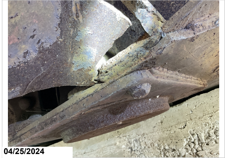
Left Railcar, Abutment 1, girder 2: 6" crack to bottom flange, and 1" vertical crack to web at Bolster
