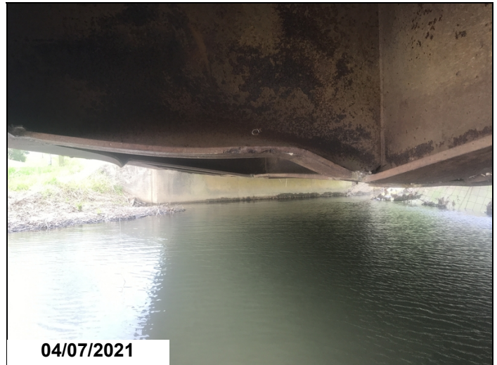
Floorbeams 1 & 2 between Girders 3 & 4 has bent bottom flange.
