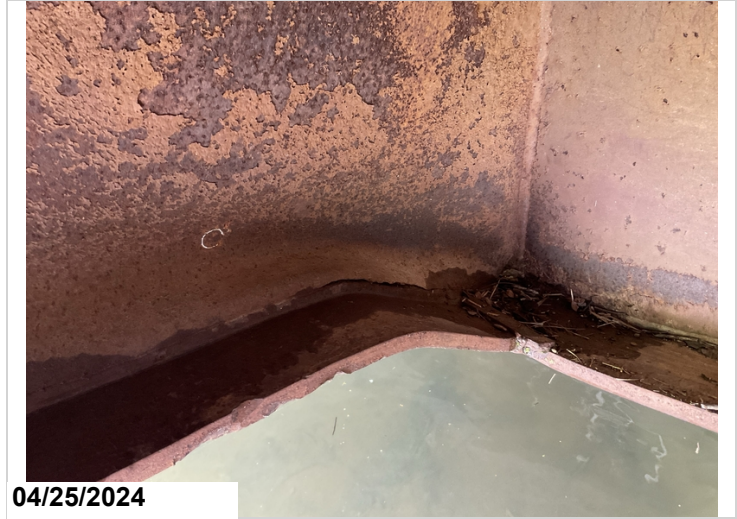
Left Railcar, Floor beam 1, Left side of Girder 2: 8" crack along the web & bottom flange connection along Floor beam.
