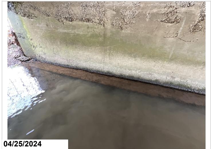
Abutment 1: footing exposed.
